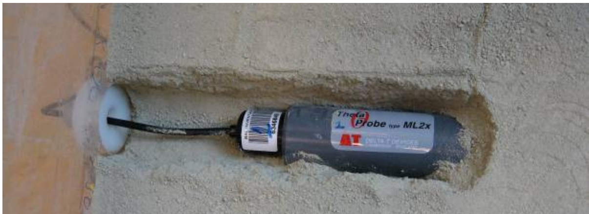
Fig. 4. Installation of the ThetaProbe (TP) sensors
